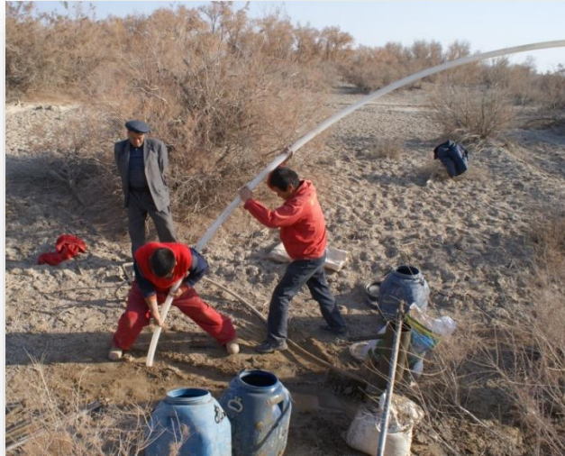
Drilling of 38 gauging stations with automatic data loggers
